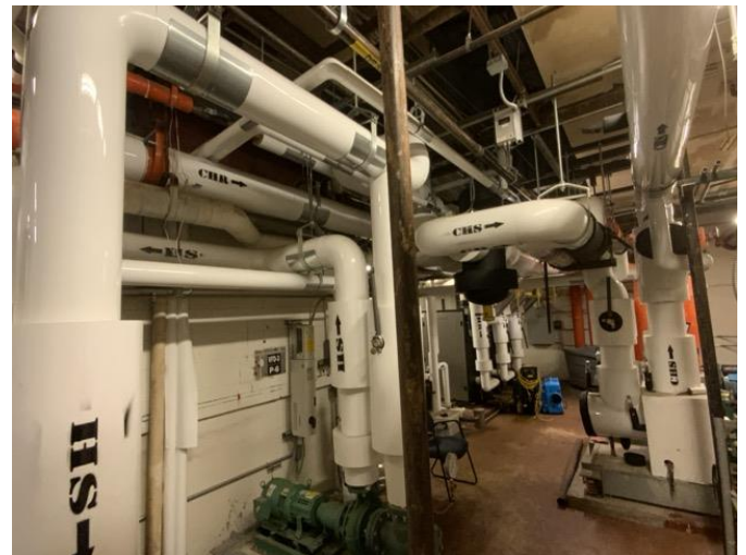
28 - HVAC HYDRONIC PIPING
