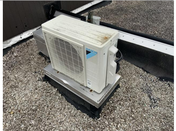
26 - SPLIT SYSTEM DUCTLESS
