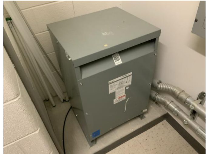
32 - SECONDARY TRANSFORMER
