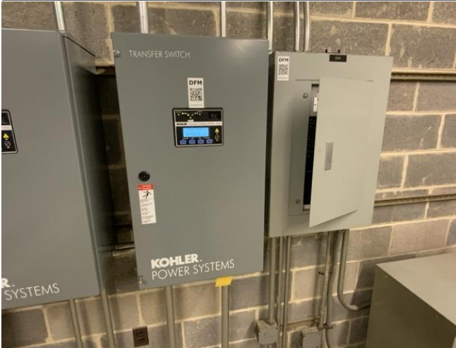
31 - AUTOMATIC TRANSFER SWITCH
